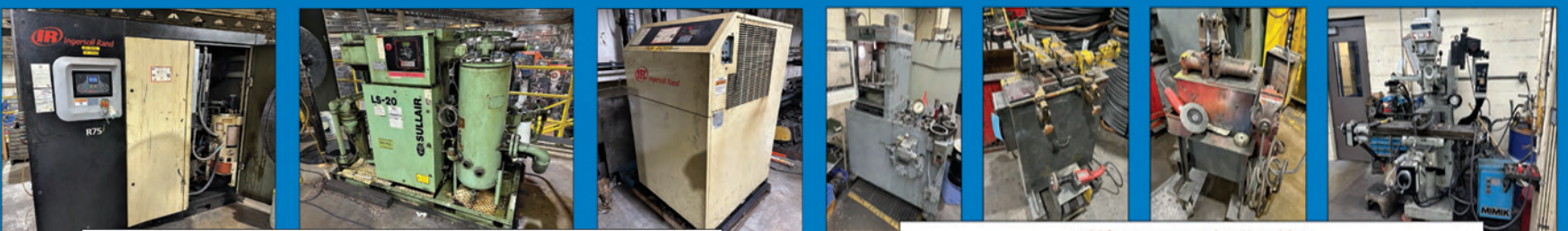
100-HP Ingersoll and Sullair Compressors
